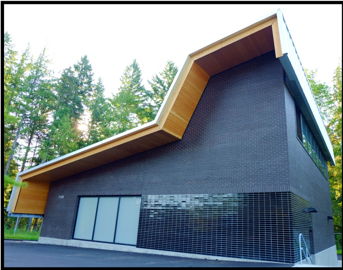
Photograph of City of Nanaimo's Reservoir #1 Energy Recovery Facility courtesy of Bill Sims, City of Nanaimo Manager of Water Resources
