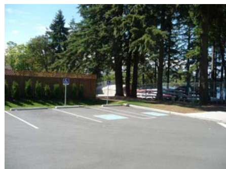
Accessible parking in new parking lot with temporary boat storage and buffer plantings visible.
