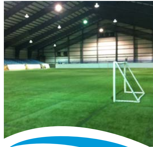
The multi-purpose Arbutus Meadows Events and Equestrian Centre in Nanaimo is 60,000 square feet with a concrete floor plus additional grounds and outbuildings.
