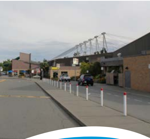
A raised sidewalk near the Social Centre helps to safely direct pedestrians through parking lot.
