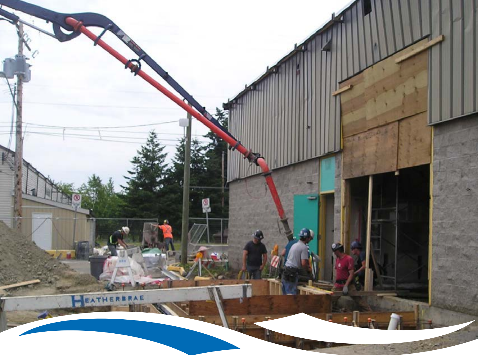
Cliff McNabb Arena renovations in progress - 2012
