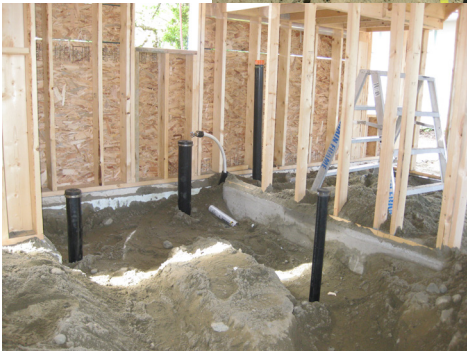
Underslab Plumbing
